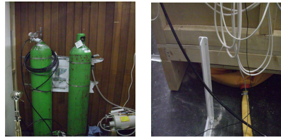
Figure 5. Compressed air and air bags
